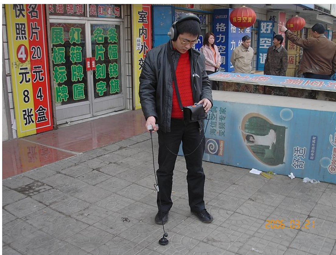
Sounding in progress
