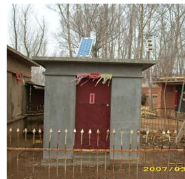
Photo : New build 'house' for new groundwater observation wells provided by the project.
